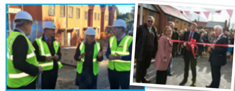
On-site at the New Queen's Head homes and opening Barron Close in Micheldever.
