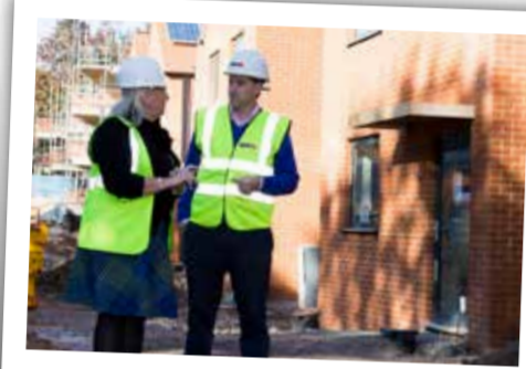
Like Conservative run Winchester City Council, Cllr Caroline Horriell and I are passionate about delivering new affordable housing in the area. Here at the New Queen's Head site in Stanmore.
